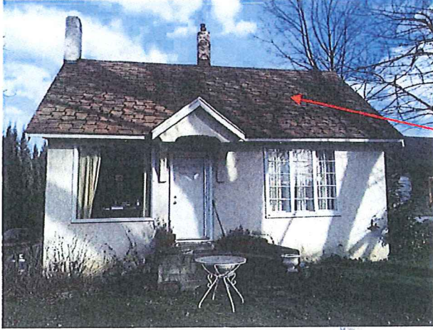
West Elevation facing Mill Creek
